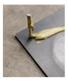
**Hollow plaques** – if plaque has a cored out back (recessed), adhere substrate (wood or rigid urethane foam) strips or blocks to plaque before you install – to help strengthen bond to mounting surface. Match substrate thickness to depth of plaque. Coat studs, stud bosses, and substrate strips with construction grade adhesive or epoxy during install.
